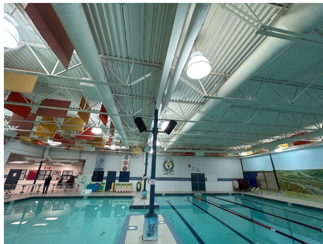
Photo 1: Existing conditions at underside of RTU location
