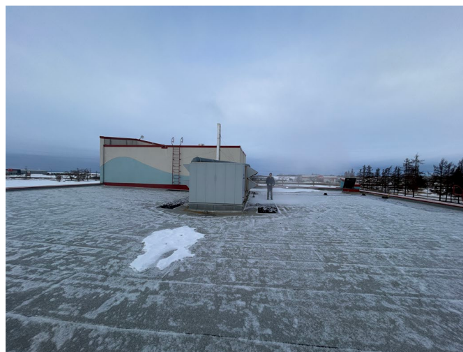
Photo 2: Existing conditions at roof topside at RTU location
