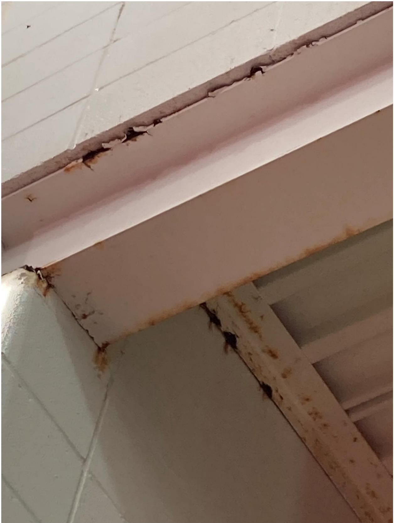
Some rust areas on the roof beams
